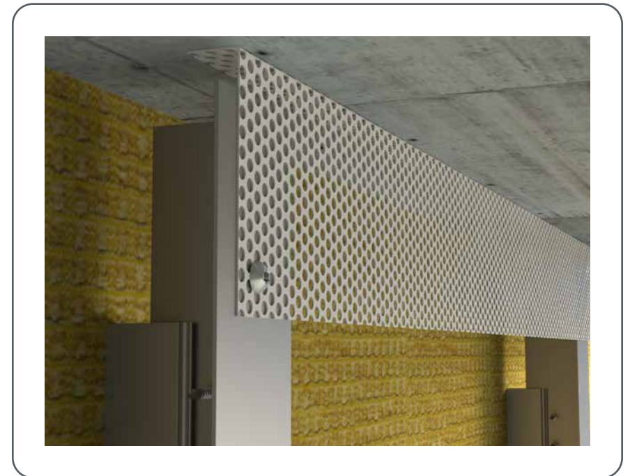
Figure 86 • Raccordement supérieur
