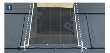
When connecting to the chimney, mark a 30 mm protrusion for the standing seam, and cut the PREFA roof covering. [1]
