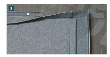
Open the top seam of the PREFA roof covering and form a lateral upstand along the marking. [3]
