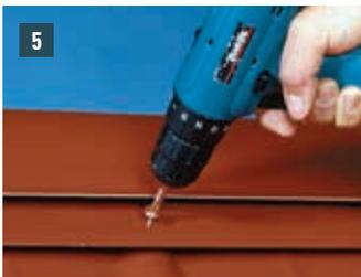
**5** Fasten the ridge vent with PREFA sealing screws (length: 60 mm) at a distance of approx. 600 mm. Note: with PREFA roof tiles, always position the sealing screw on the crest. With roof shingles and roof tiles, do not screw onto the inclined hook seam. With R.16 roof tiles and FX.12 roof panels, do not screw onto the vertical standing seam.
