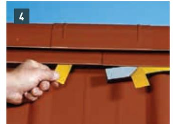
**4** Glue the sealing wedge (with the sealing surface already stripped off) under the connection sleeve. Then carefully remove the protective film.
