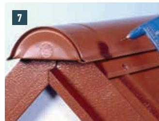
**7** Adjust the ridge vent end cap and attach with a rivet.
