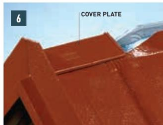
**6** Suggestion for installing the ridge vent end cap: first mount the cover plate in the edge area and form a 30-mm upstand for the verge flashing. Then mount the verge flashing.
