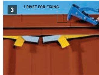
**3** Fit both connection sleeves in the centre and use a PREFA rivet ( $\varnothing$  4.1 mm) to fix each one in place.
