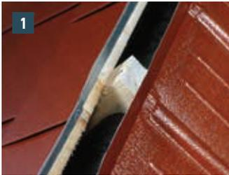
**1** The last row should be oriented such that an air gap of 80 mm is created. Position the PREFA roof elements approx. 40 mm vertically.
