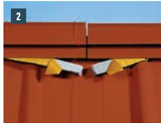
**2** Observe expansion joints of approx. 5 mm between the individual ridge vents, remove approx. 50 mm of the protective film from the sealing wedge and bend outwards.
